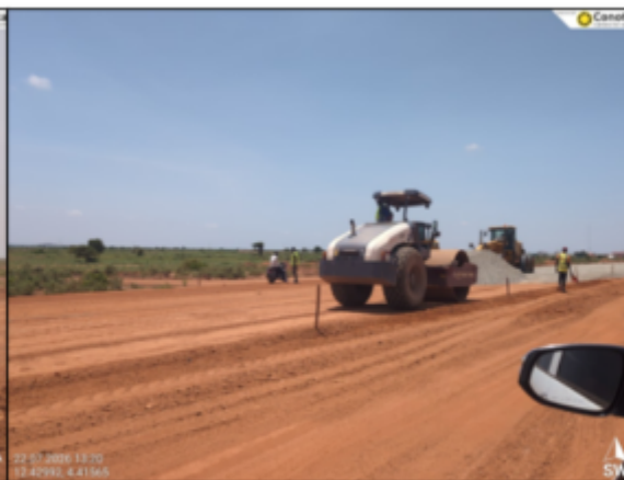
Photo 8: A single-drum roller compacts the subgrade of a new road formation
