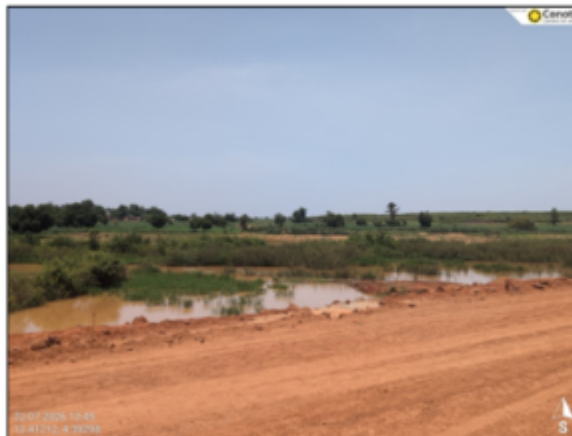
Photo 4: Standing turbid water in shallow depressions immediately adjacent to the earthworks
