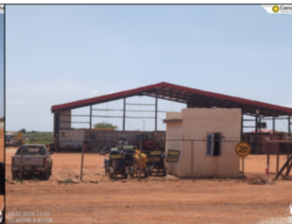
Photo 9: Steel-framed building stands over stored plant and equipment
