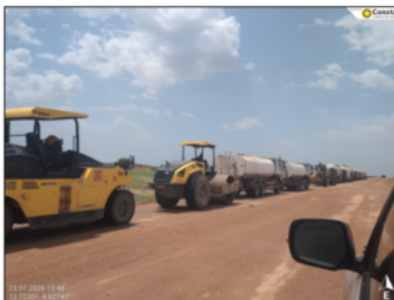
Photo 16: A line of parked construction plant along the edge of a haul road
