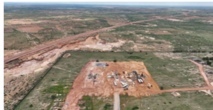
An Aerial imagery of the batching plant along CH 144
