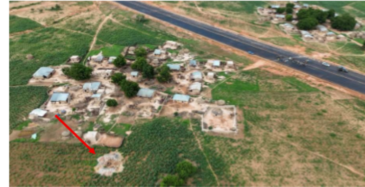
An Aerial imagery of the distance of the temporary palliative well dug for the Lagga Gidan Namata Community
