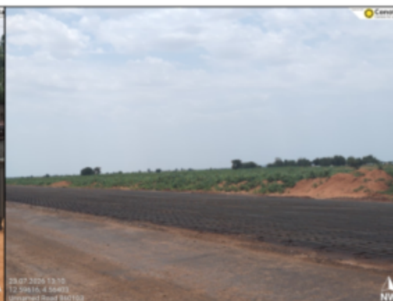
Photo 15: A newly formed road embankment
