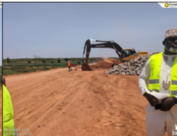
Photo 5: Excavator digging up sand
