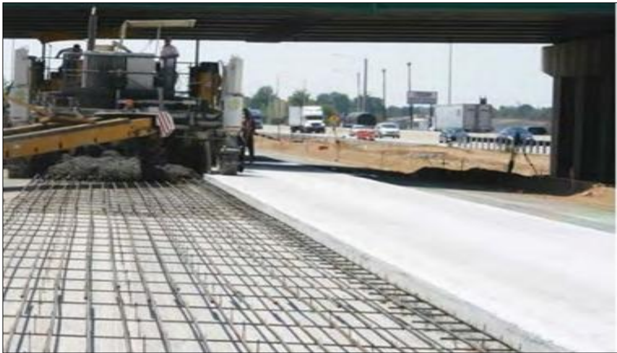
Plate 3.1: Typical CRCP Laying Procedure
