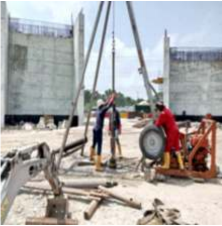
Hitech Geotechnical team carrying out soil investigation with the Dando III Percussion drilling rig. Location: REGIONAL ROAD PROJECT VGC LAGOS
