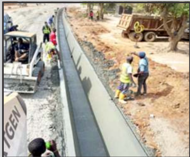
PIC3: SLIPFORM TRAPEZOIDAL DRAIN
