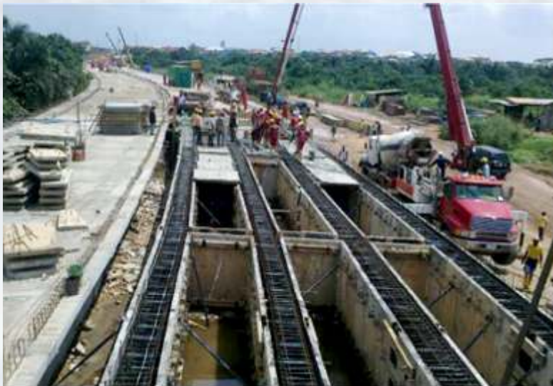
Isheri Oshun, Alimosho Local Government, Lagos flyover under construction
