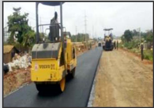
PIC 1: LAY 60MM ASPHALTIC BINDER
