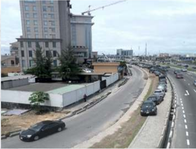
Ozumba Mbadiwe road under construction
