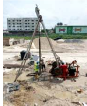
Hitech Geotechnical team carrying out soil investigation with the Dando III Percussion drilling rig. Location: REGIONAL ROAD PROJECT VGC LAGOS
