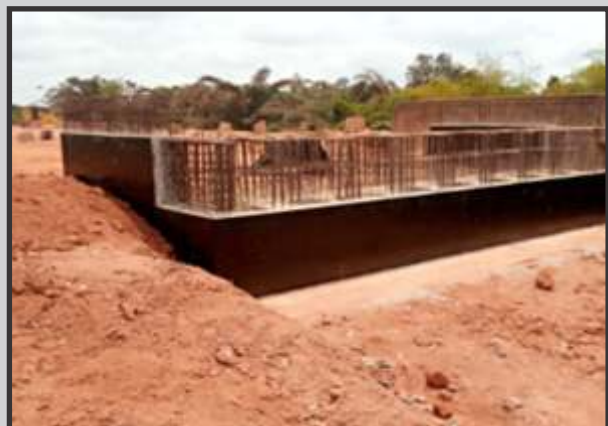
PIC4: WADI BRIDGE EXIT ABUTMENT
