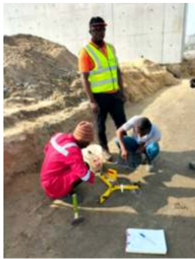
AEC consultant road supervising field density test
