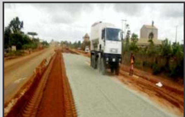
PIC2: SUBBASE STABILIZATION PROCESS
